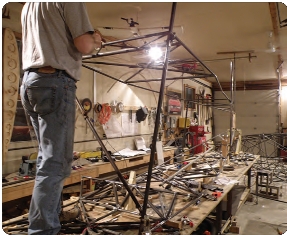
The plane under construction.
