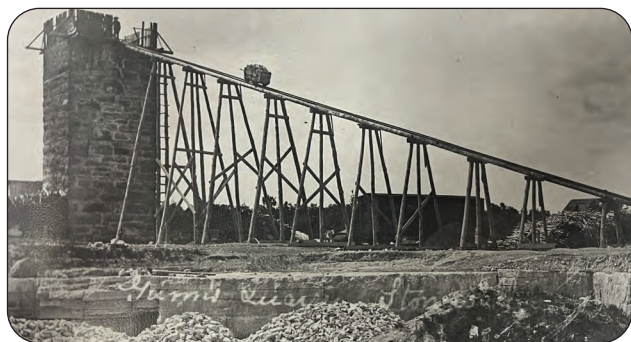
THE GUNN QUARRY - This kiln, located in the Gunn Quarry (South-East), was first fired in May 1900. The trestle, on which cars of rock were drawn up, was built by Andrew Mitchell.
