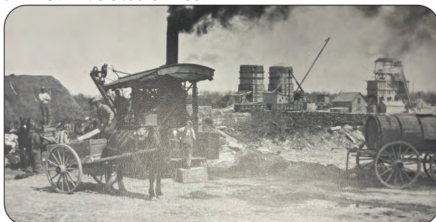
QUARRY EXCAVATION - This steam excavator was used to clear the top soil from the rock. Archie Billings operated the excavator for many years.
