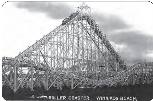
The historic wood roller coaster in Winnipeg Beach, 1927.
