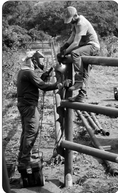
Drysdale and Scott Blais welded steel rails to five- and six-inch poles.
