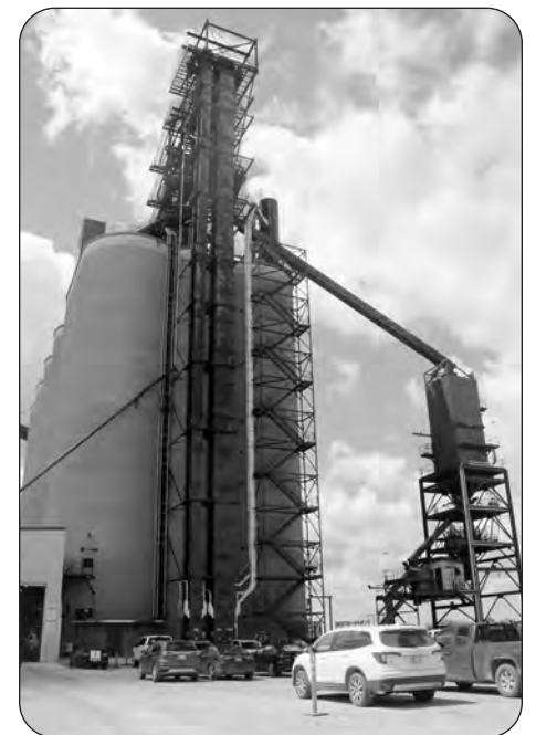
The facility has the capacity to load 156 rail cars during a 12-hour period.
