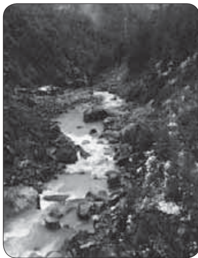
The river below the suspension bridge.
