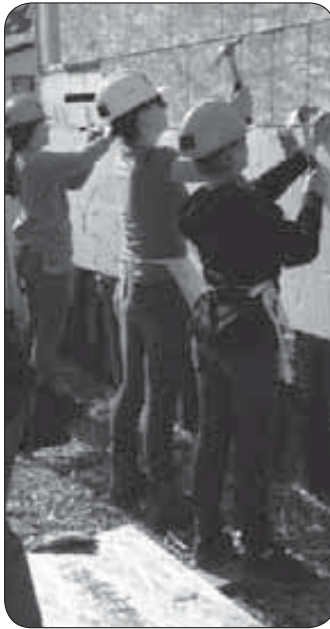
A group of SCI students watch and learn from one of the crew members as he shows them how to fasten wood sheathing to a side of the house.
