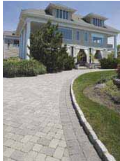
Choosing the right paving materials can add instant character to your yard.
